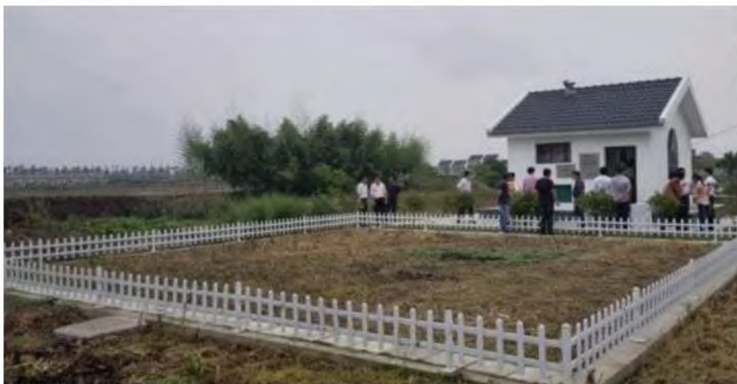
No.5 wastewater treatment station, Damang village, Shanghai
