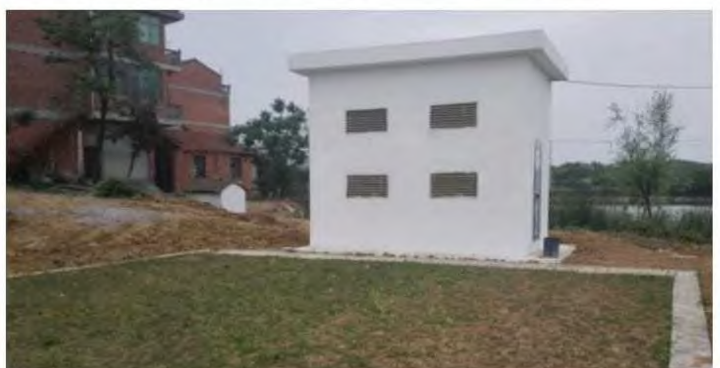
Xidian village wastewater treatment station, Yiwu City, Zhejiang Province
