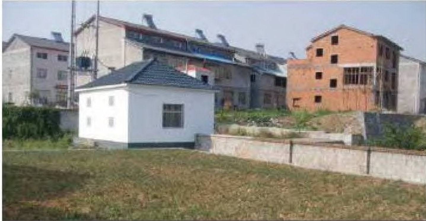
Guangzhuang village wastewater treatment station, Yichang City, Hubei Province
