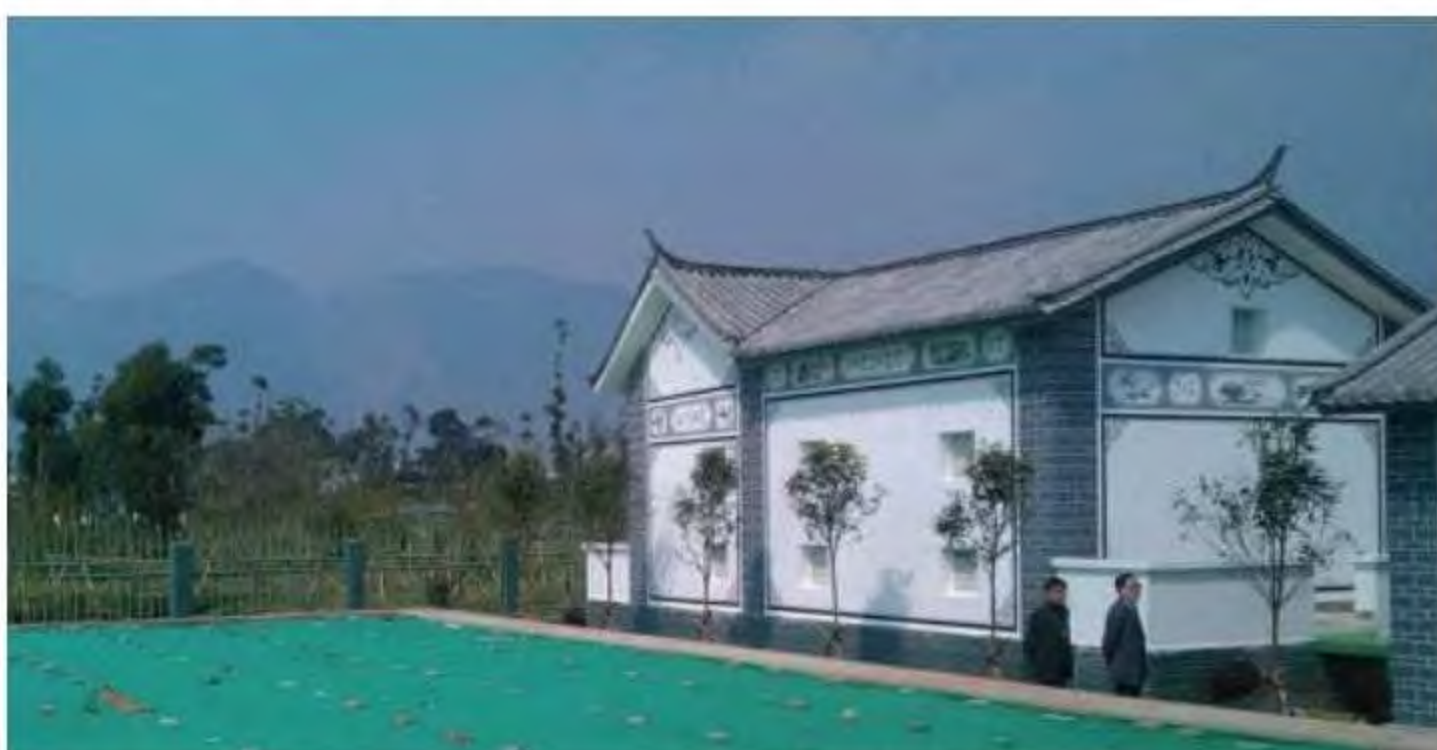
Geguanying village wastewater treatment station, Eryuan County, Yunnan Province
