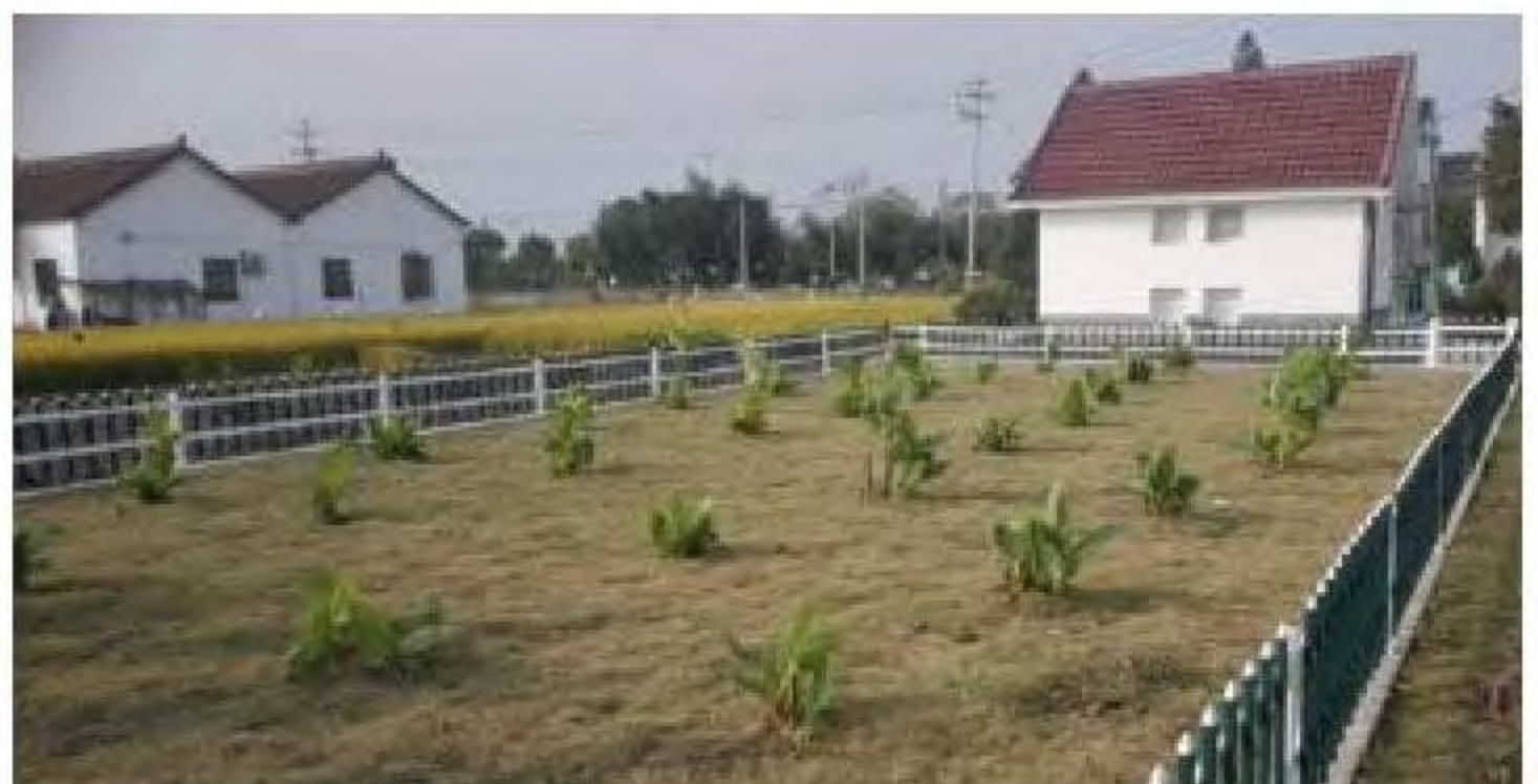
Yujiadai village wastewater treatment station, Huzhou City, Zhejiang Province
