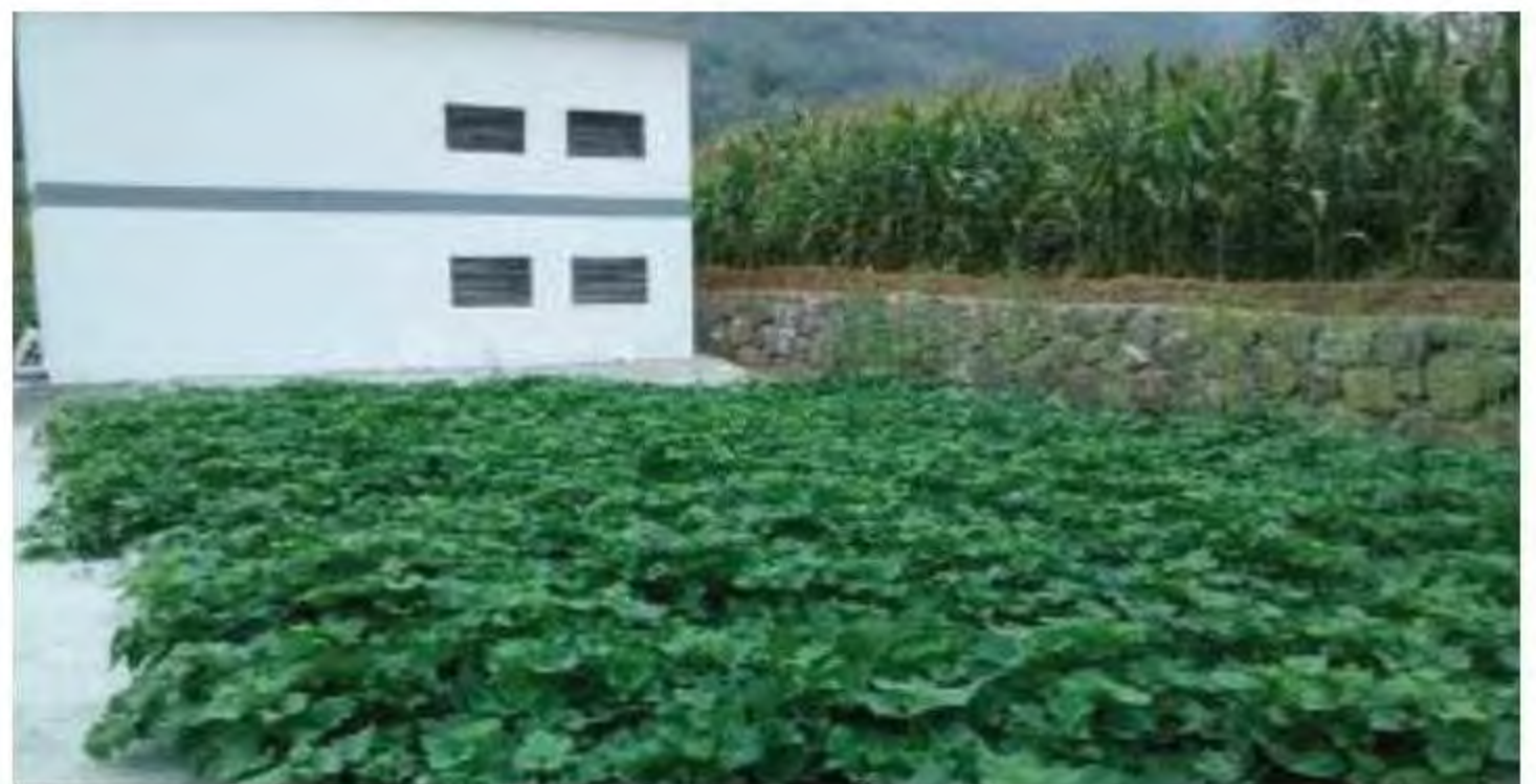
Xiachangping village wastewater treatment station, Xiangshan County, Hubei Province
